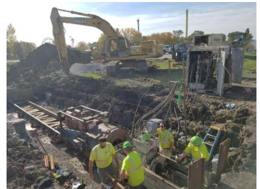
30" Storm Sewer Bore Under Hubbell Ave
