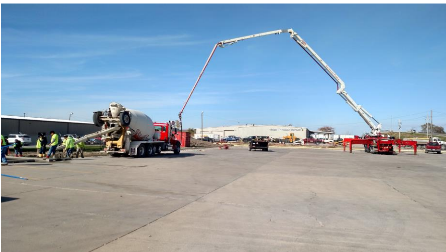
Paving the Expanded Parking Lot at Quality Trailer on October 25
