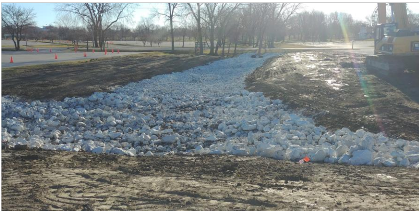
Storm Outlet at Adventureland Park
