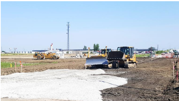
Elder placing granular base before paving operations
