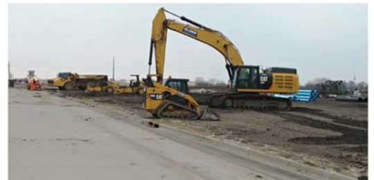
Equipment Waiting and Ready to Go
