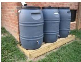
Rain barrels collect and store rainwater from rooftops for watering lawns and gardens. The water captured reduces the amount of stormwater running off the property during rainfall events. Because this water is not treated, it should not be used for drinking water.
